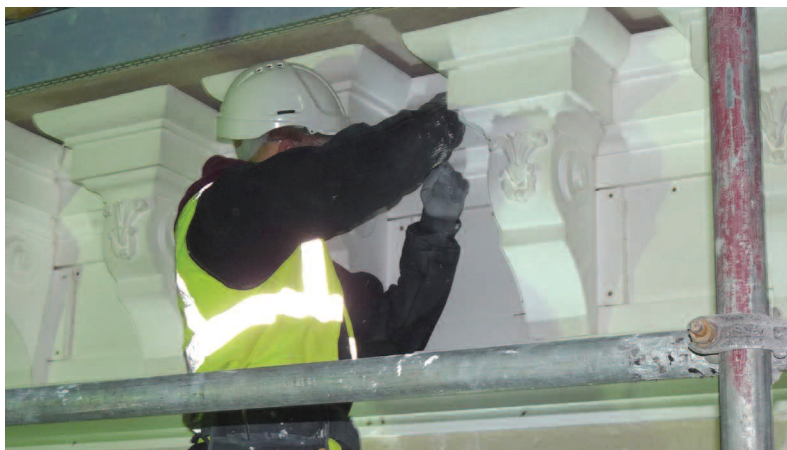
Jake in action. An example of the scale of size of the corbels fitted.
