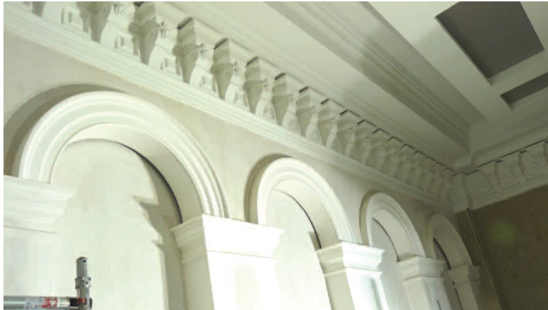
Three-coat sand lime plasterwork to walls, semi-circular arch head and plaster head mouldings to match existing.
