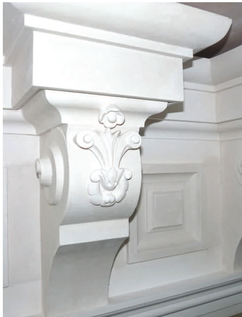
New corbels that were fitted, although not fitted direct to the ceiling for acoustic reasons.
