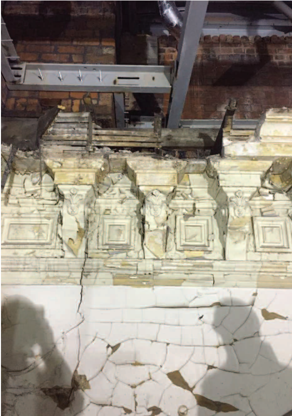
Original details to replicate from. All had to be removed due to rotten timbers.
