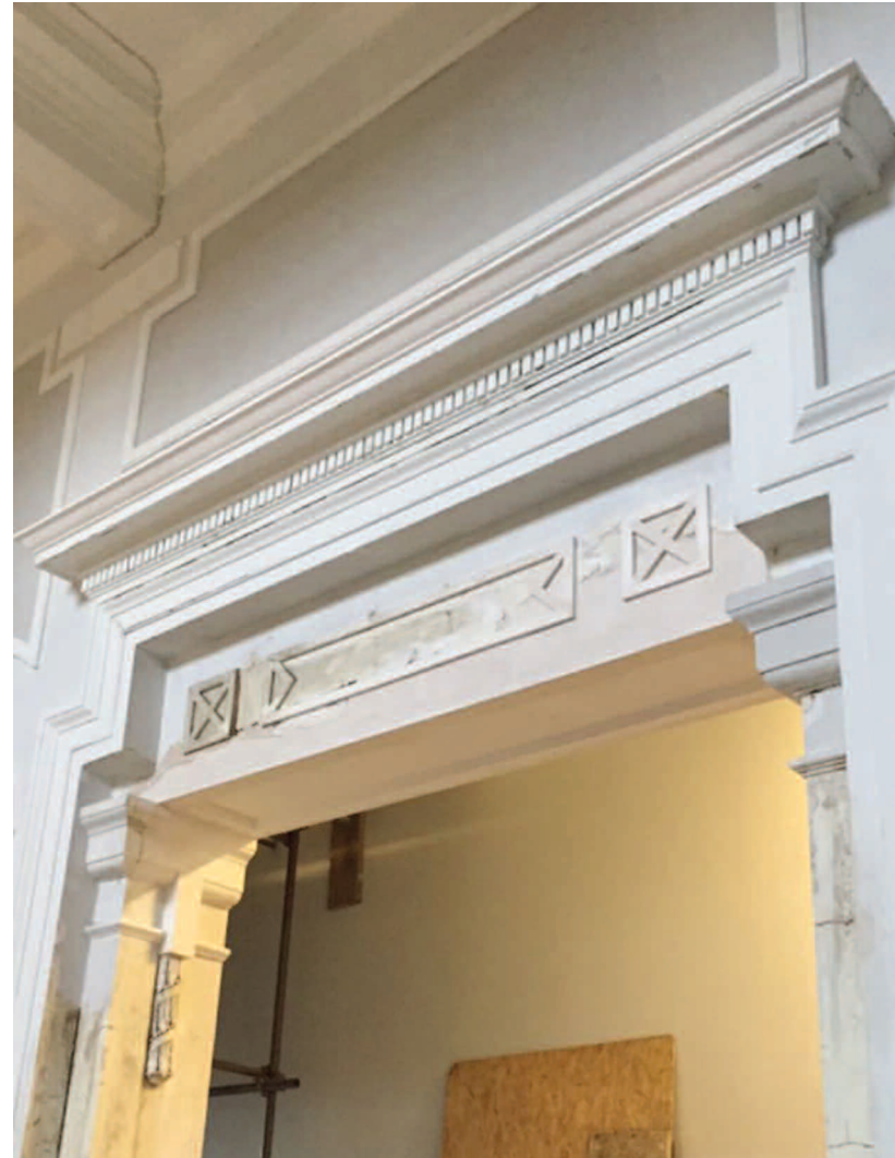
Before and after of the restored lintel details and pilaster caps on doorway to cinemas on staircase two.
