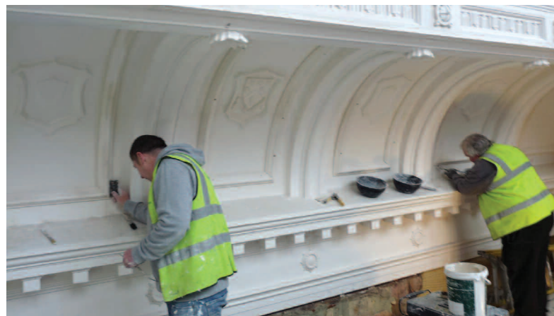
Ian and Ray putting final touches to panel mouldings.
