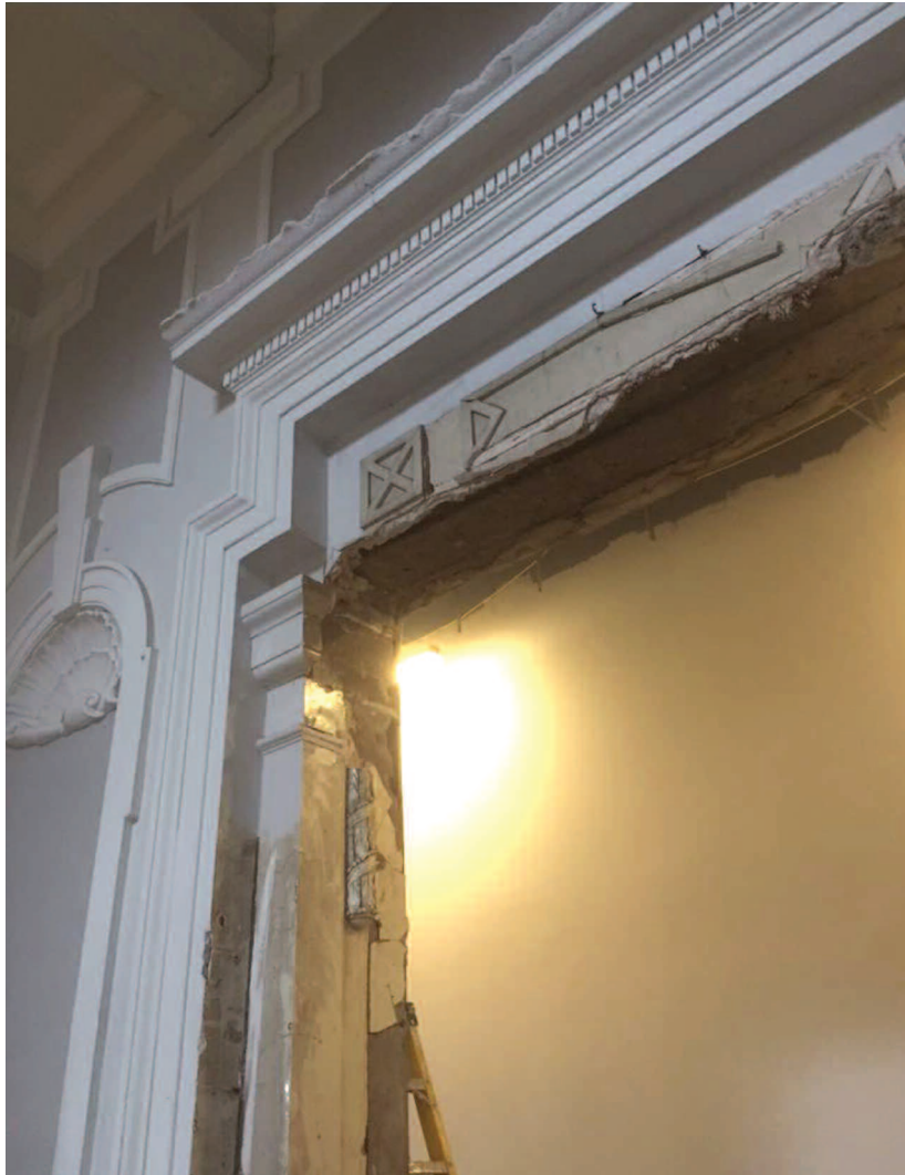
Before and after of the restored lintel details and pilaster caps on doorway to cinemas on staircase two.
