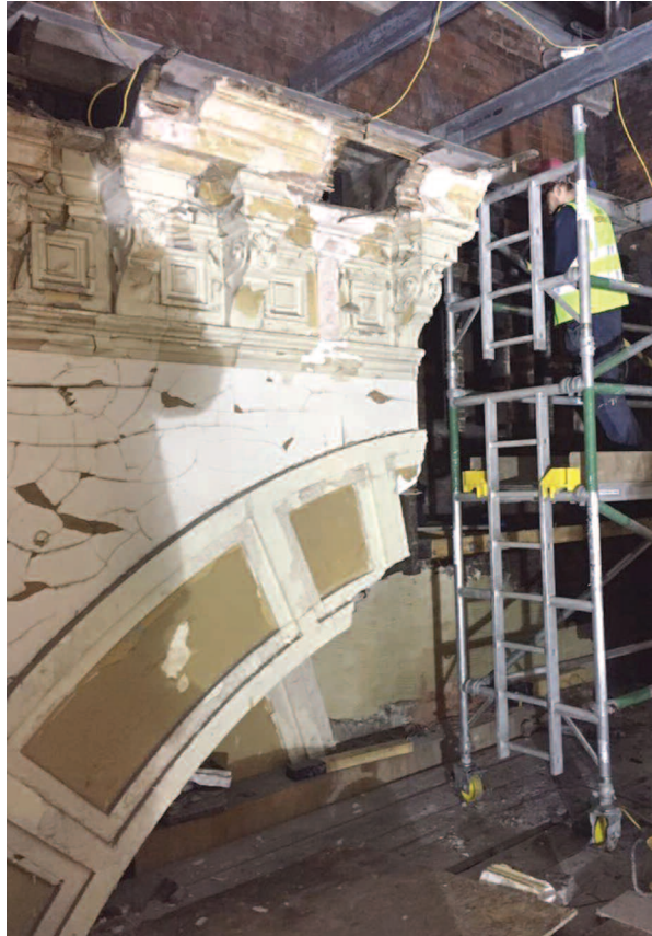
Original details to replicate from. All had to be removed due to rotten timbers.
