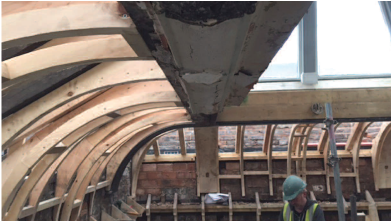
Elements that were existing couldn't be used due to rotten timbers.
