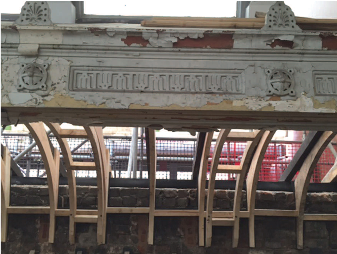
Replaced rotten timbers before we started work
