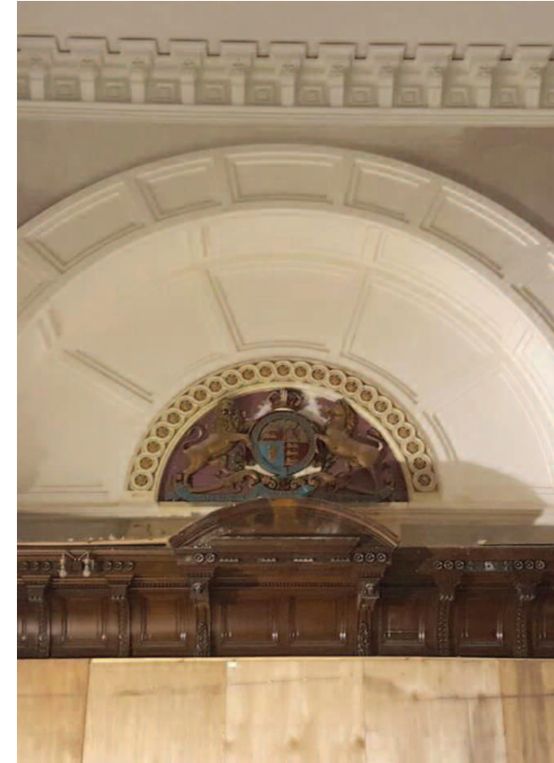
New proscenium arch and restored crest installed.
