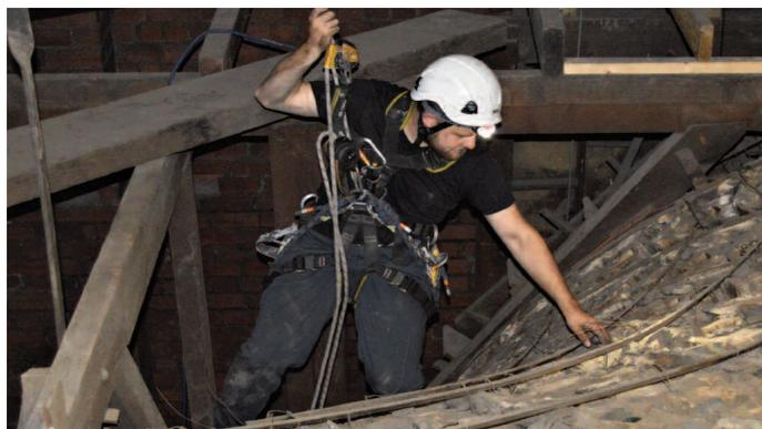
Paul from Ormate Interiors checking 1878 open fret work cast plaster panels forming Gothic Fan Vaults at the corners of theatre ceiling
